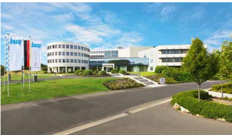
Knauf Main Administration in Iphofen (Germany).
